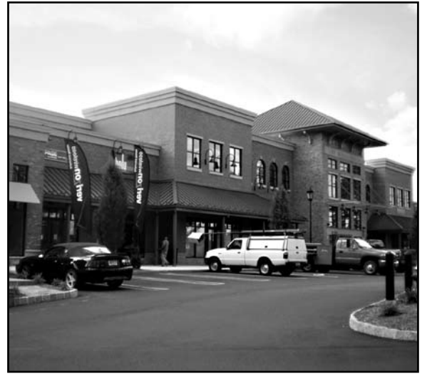
100 Marketplace is a 57,600 square-foot mixed-use project located in Basking Ridge, N.J., and financed by David Cronheim Mortgage earlier this year. Photo courtesy of David Cronheim Mortgage.
